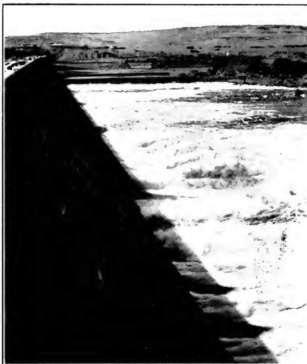
THE SLUICES OPENED AT ASSUAN TO RELEASE EXCESS WATER FROM THE RESERVOIR ABOVE
